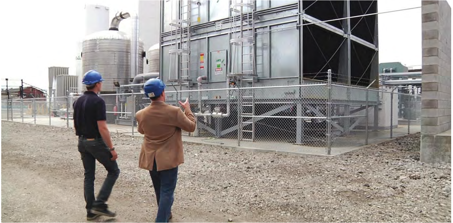
Voltea personnel observe the cooling towers on-site at Republic Steel.
